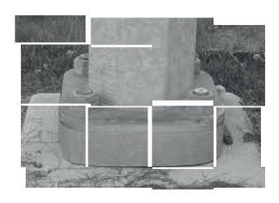
High compressive strength and density combined with low absorption are important to the long-term durability of the concrete. Lower-quality concrete can deteriorate in under a decade due to the aggressive environment that the roofs and the ballasts create.
